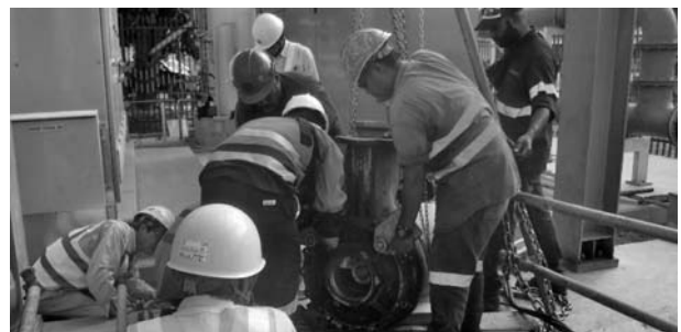
Photo. 2 Operation and Maintenance Training
