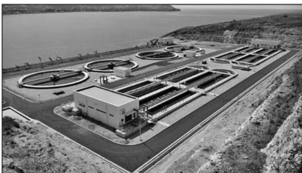
Photo. 1 Sewage Treatment Plant Panoramic View
