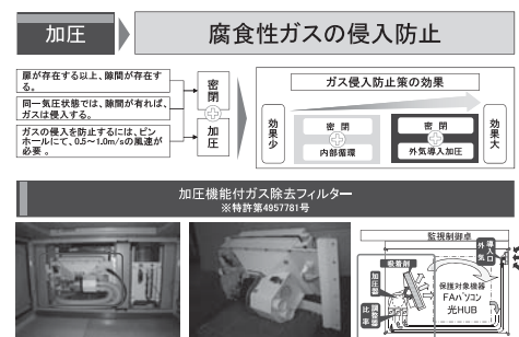
Fig. 2 A corrosiveness gas removal filter unit with a pressurization function
