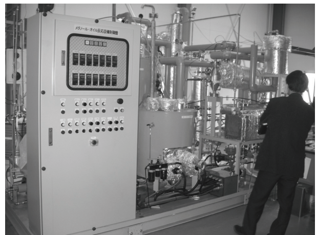
Fig. 3 Pilot-scale reactor which can produce 40 L of fatty acid methyl ester based on super-heated methanol vapor method.
