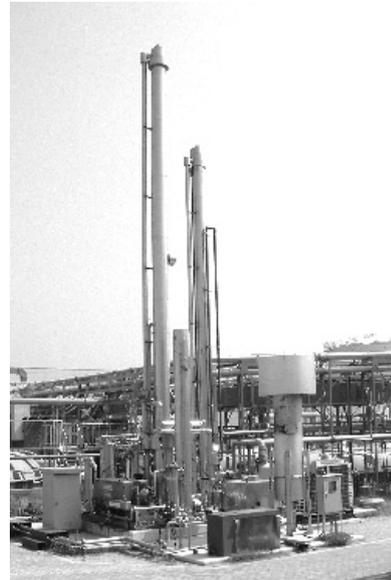
Fig.3 Overview of biogas purification demonstration plant
