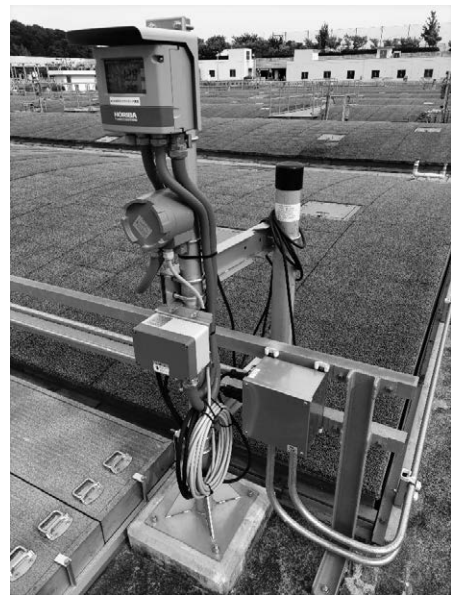
Photo. 1 Installed ammonia meter
