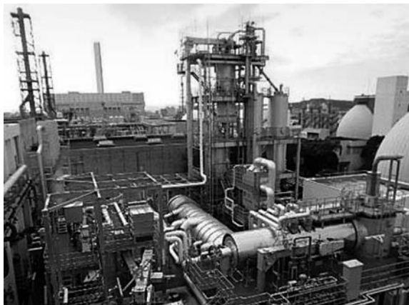
Photo. 1 View of sludge to fuel conversion facilities
