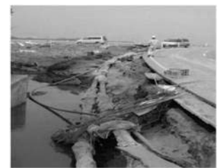
Photo. 2 There is no damage of the earthquake-resistant pipe after the tsunami (Japan Ductile Iron Pipe Association)
