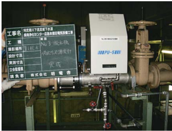
Photo. 5.7 Restoration status of supplied-sludge density meter for No. 3 dehydrator (Photo taken in Oct. 2011) The equipment in the No. 1 dehydrator building was the first to be restored.
