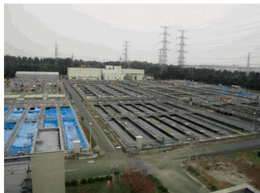
Photo. 3.6 The water treatment facilities (Photo taken in Nov. 2011)
