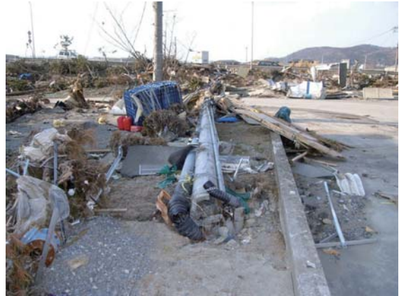
Photo. 2.8 The destroyed NTT (Nippon Telegraph and Telephone Corporation) service leading-in pole (Photo taken by staff member at the STP in Mar. 2011) The power receiving wire pole was destroyed by the Tsunami.
