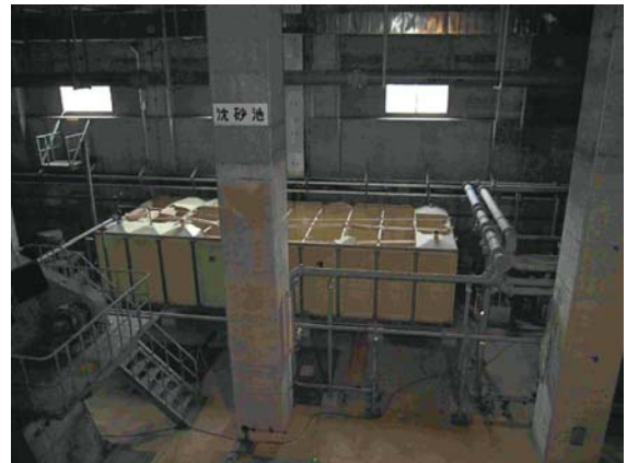
Above : Immediately after the Tsunami. Submerged in water because it was installed on the basement floor. (Photo taken by staff member at the STP in Mar. 2011) Below : Under restoration work after water was drained (Photo taken in Nov. 2011)
