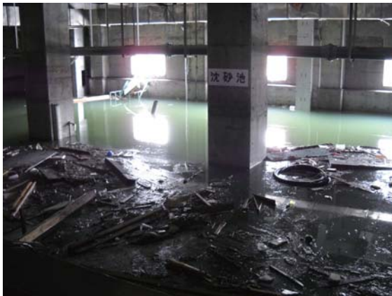
Above : Immediately after the Tsunami. Submerged in water because it was installed on the basement floor. (Photo taken by staff member at the STP in Mar. 2011) Below : Under restoration work after water was drained (Photo taken in Nov. 2011)
