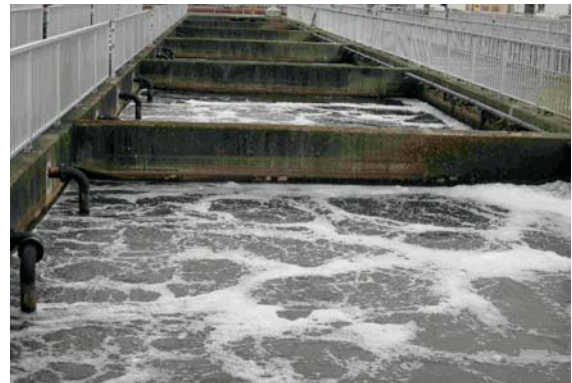
Photo. 3.11 Simple aeration (Photo taken in Nov. 2011) Simple aeration, that means aeration without return sludge, was performed temporarily
