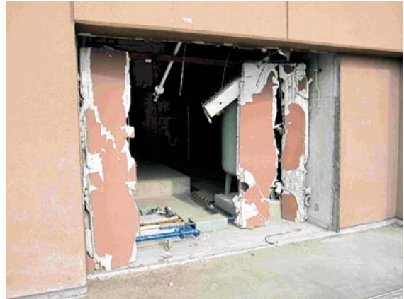
Photo. 2.5 Equipment carry-in entrance on the 2nd floor (Photo taken in Nov. 2011)
